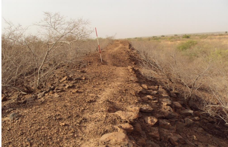
Fig. 2: The Defensive wall at Surame (Source: Department of Archaeology and Heritage Studies, ABU Zaria 2012)
